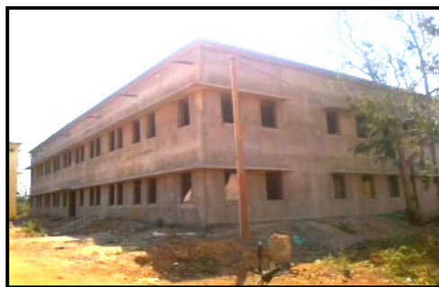
Construction of barrack at CPMF Headquarters, Koraput with RCC roof
