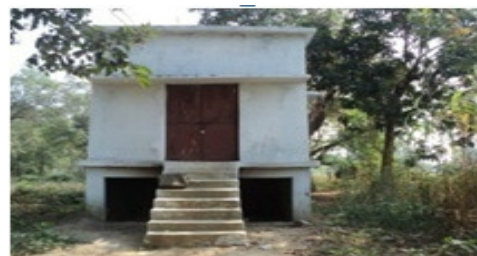
Photograph of RPWS at Janged in Bargarh district which remained non functional due to non completion of electrification works
