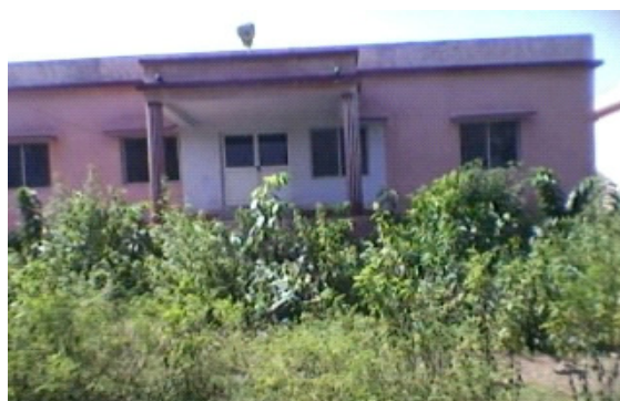
Non-functional CHC building at Boipariguda
