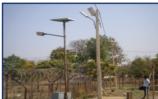
Installation of lighting system at Meghpal ANPP, Sambalpur without power supply
