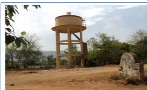
Elevated storage reservoir of RPWS to Makarsola in Kalahandi district without pump house and external electrification works
